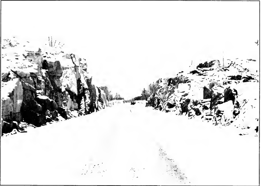
Rock Cut, Highway No. 7, 5.3 Miles East of Marmora.
